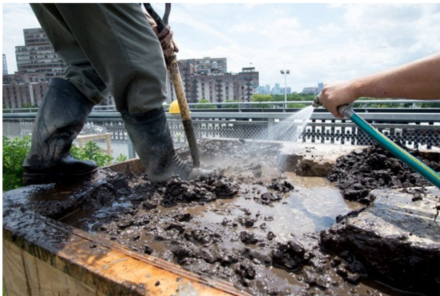
The installation in progress. Timothy Schenck
