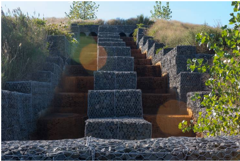
A drainage structure at the former Fresh Kills Land Fill in Staten Island, which was once the largest garbage dump in the world and is being transformed into a park. PHOTO: MANSURA KHANAM FOR THE WALL STREET JOURNAL
